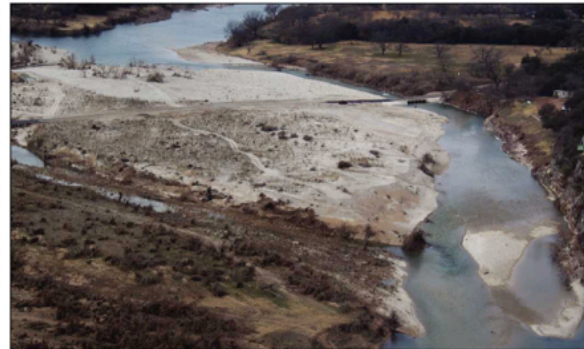
James River Crossing following October 16, 2018 flood
