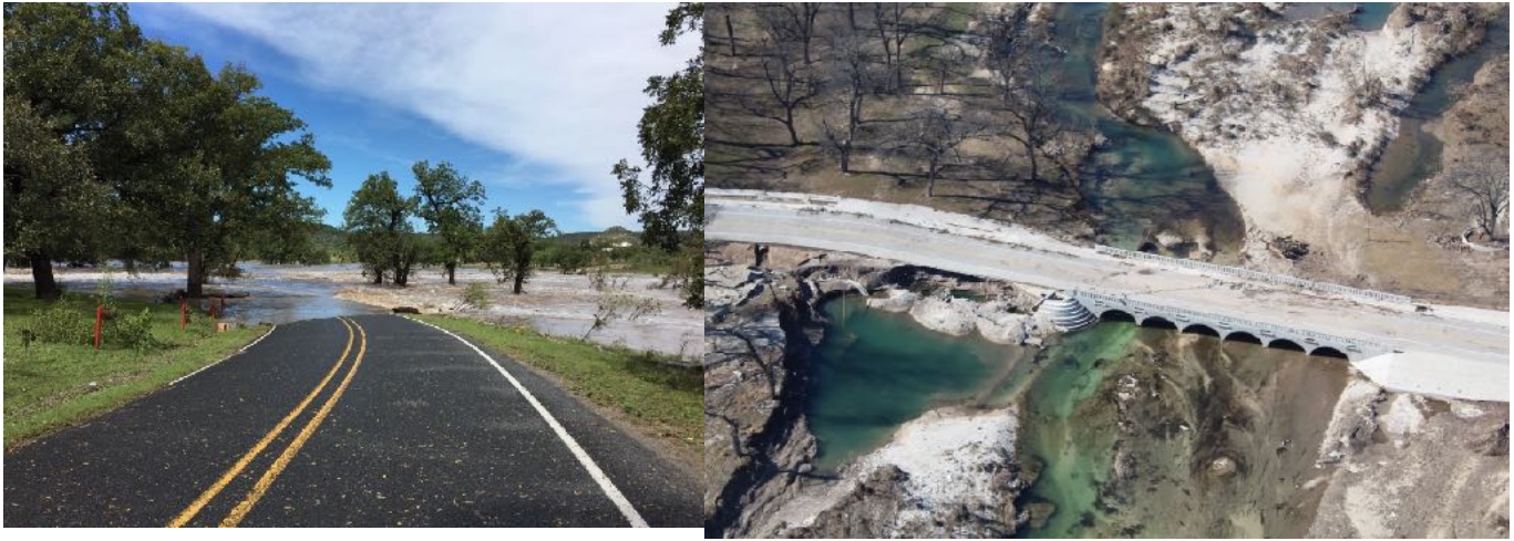
Figure 14. Left: Southern approach to Flat Rock Bridge near Junction - October 9, 2018. Right: Aerial view of Flat Rock Bridge looking west - December 14, 2018
